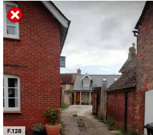
Figure 127: The Cedars, left, and Badger House, right, are an example of unsympathetic infill redevelopment and good restoration at the Badger crossroads (Source: Blandford Plus NP Steering Group)
