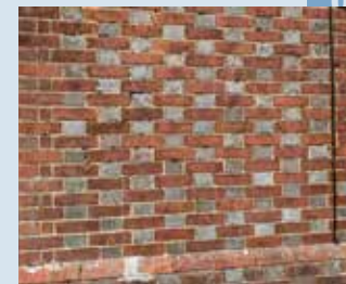
Brickwork in Flemish Bond
